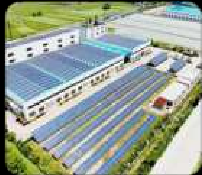
Product: Three-phase 30kW Project Size: 2.0MW
